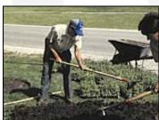
Apply compost by hand, using rakes or shovels, or mechanically with a front-end loader, grading blade, manure spreader, York rake, or other appropriate equipment
